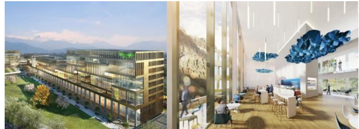
Campus GreenOValley, Schneider Electric, Grenoble
